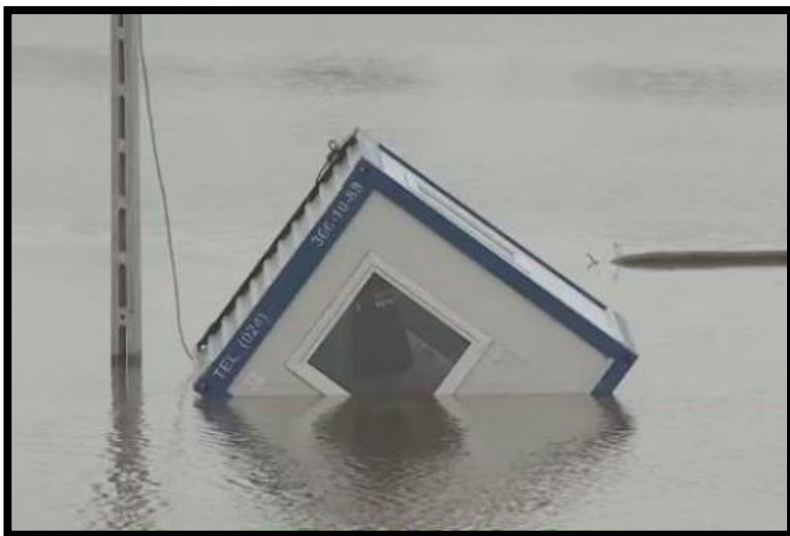
Flood affecting A1 motorway construction site
